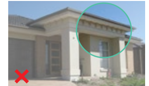
Eave brackets not allowed
