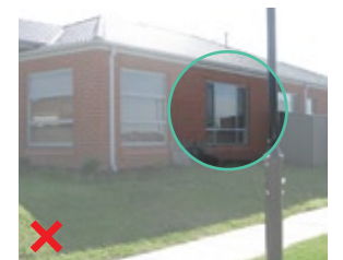
Side street window does not match style of front windows
