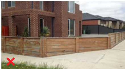
Front fence not transparent and does not compliment the style and colour of the home
